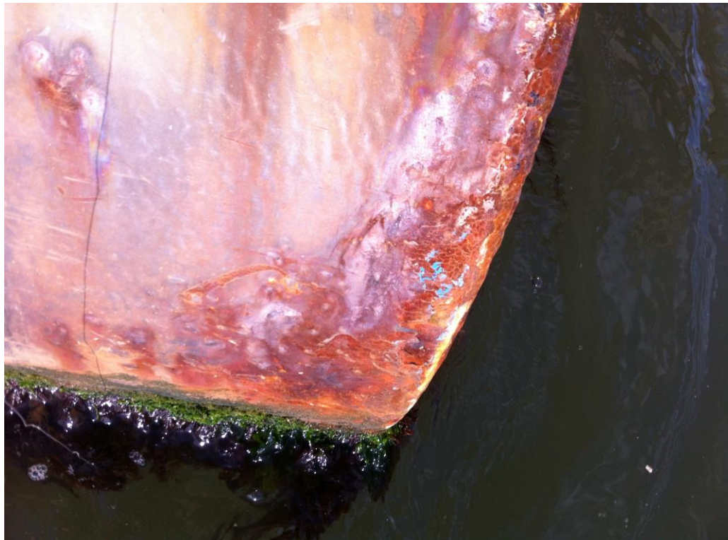
30m Pontoon Outer Tube North - Weld Pitting & Corrosion
